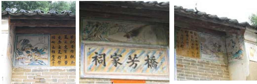
Decorative Features and Name of Building above Lintel
