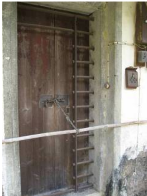
Granite Doorways with Iron Bars and Blocked Arch Opening at Side Wall
