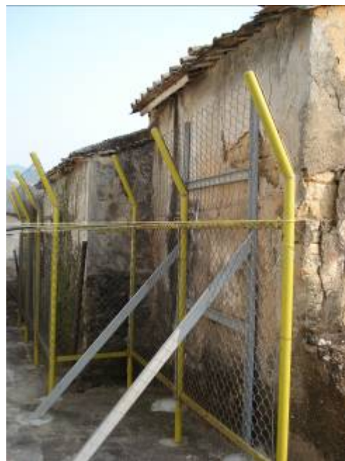
Back View (With External Structural Support)
