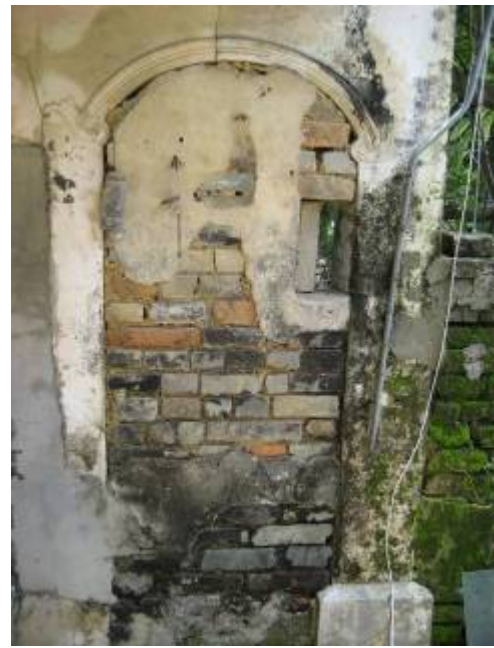
Granite Doorways with Iron Bars and Blocked Arch Opening at Side Wall
