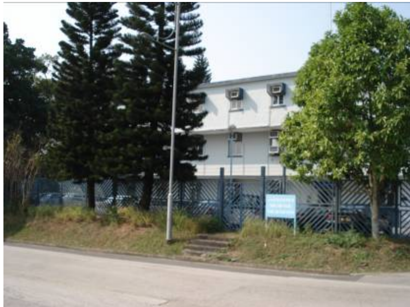
Side View of the Police Station
