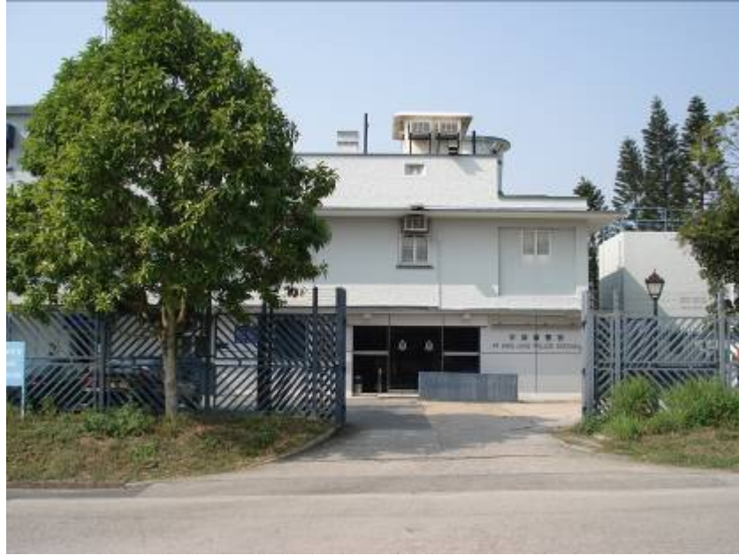
General View of the Front Gate of the Police Station
