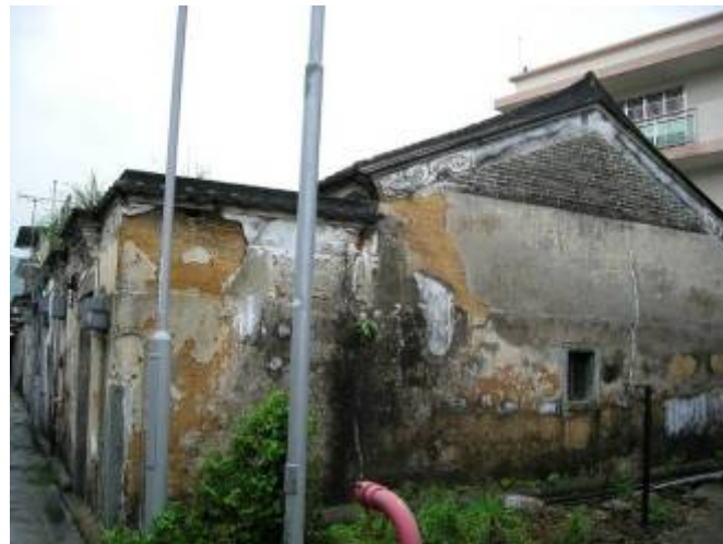
West Side Wall with Window Opening
