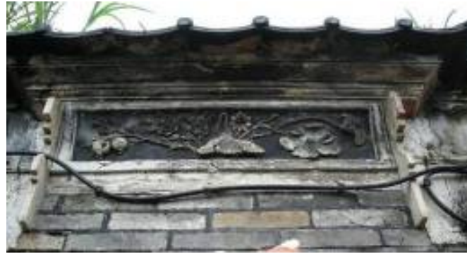
Façade Wall Frieze Decorative Feature of the First Bay from the Easternmost End
